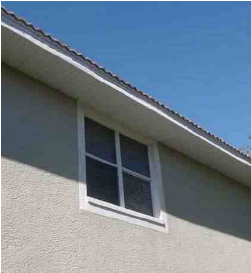
Unprotected Opening
